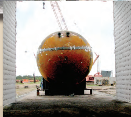
112' long section of a 17' I.D. x 203' long tank ready for PWHT
